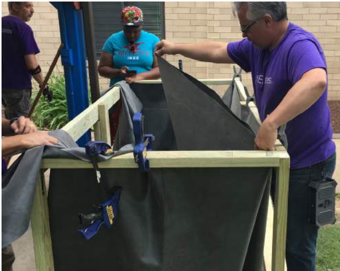
FedEx Ground volunteers attach a pond liner material to the frame.
