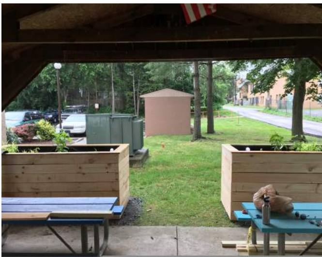
Two completed flow-through planter boxes.
