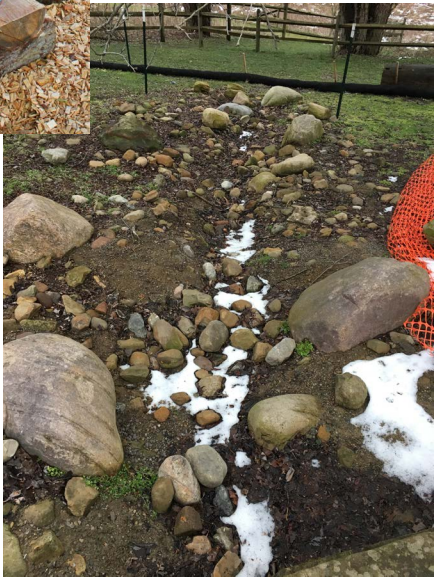
Stream enhanced with a variety of stone sizes
