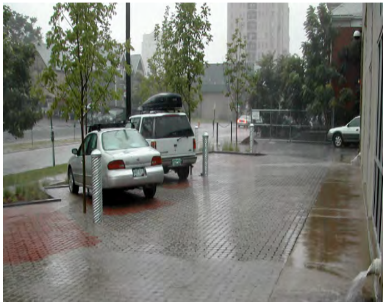
A porous paver parking lot absorbing roof runoff. Photo courtesy of Wenk Associates.
